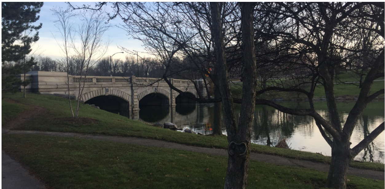
Lincoln Parkway Bridge in Delaware Park, part of the Buffalo Olmsted park system.
