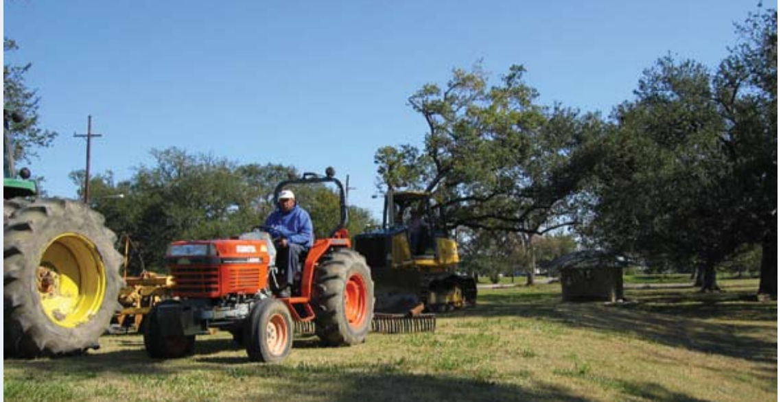
Boh Bros. construction equipment is a welcome sight in City Park.
